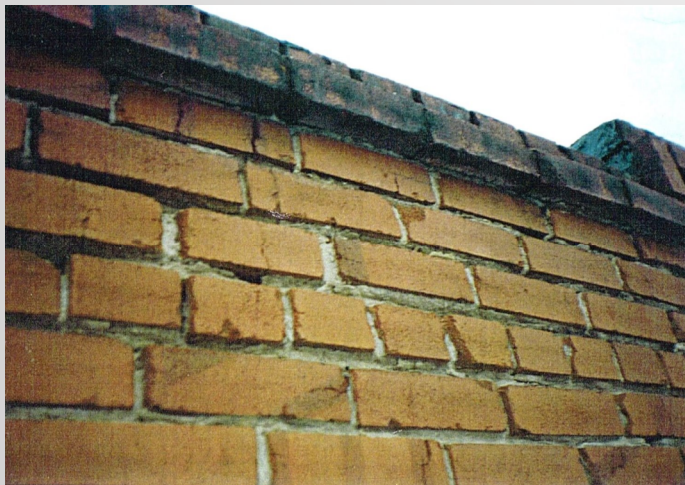
Figure 4 – Adjacent parapet wall
