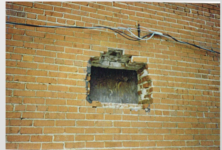
Figure 5 – Adjacent parapet wall
